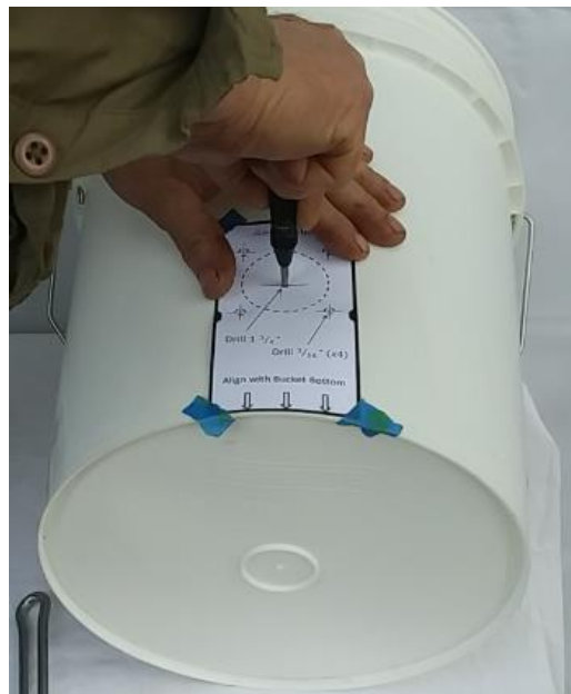
Figure 3 Locate holes.
