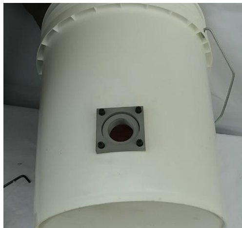
Figure 7 Install outer bracket.
